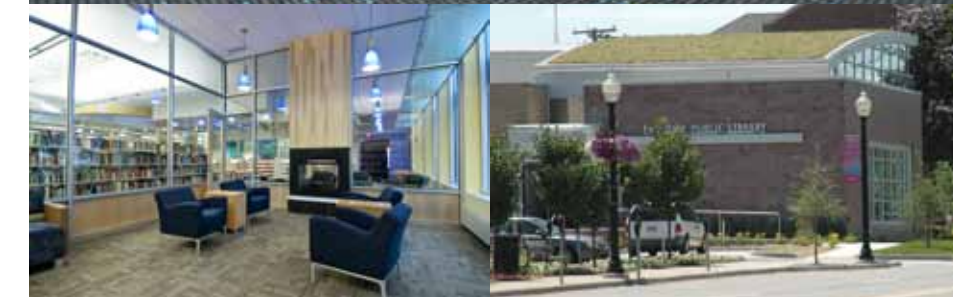
Colorful and spacious public areas, a computer lab, and expansive low-e reflective glass windows help make the Ferndale Public Library both a delight to visit and an extraordinary example of leading-edge energy-efficient architecture and construction.
